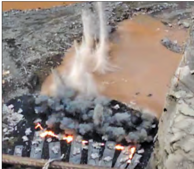
Barrier blasting at Baglihar Hydroelectric Project, Stage-II (J&K)
